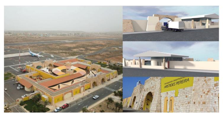
The new Cargo Terminal is formed by a perimeter wall built of concrete walls and rectangular concrete block walls enclosing a covered central area, which acts as a loading and unloading dock and offices, and two covered side areas for offices, maintenance and warehouse.
